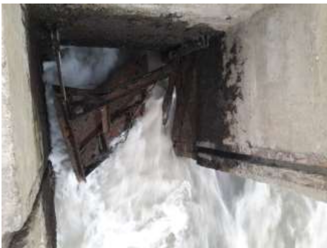
Fully nonfunctional sluice gate in Sobaki (22.572338, 89.779705).
