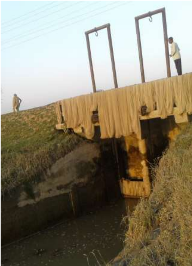
Poorly functioning Sluicagate in the Par Batiaghata (22.729765, 89.468265)
