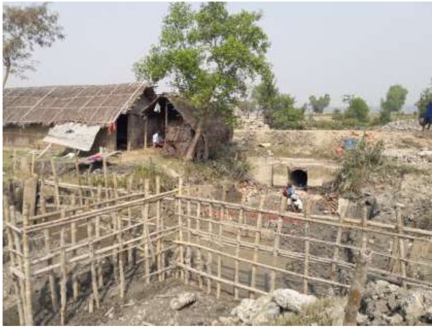
People are building drainage inlet by cutting embankment themselves
