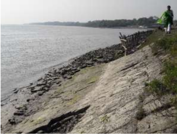
Polder line erosion beside Batiaghata bazar (22.732960, 89.518741) and near Ferry ghat bazar (22.633342, 89.520384) in Kajibacha River.
