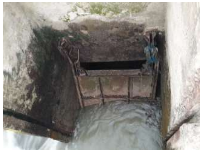
Fully nonfunctional sluice gate in Sobaki (22.572338, 89.779705).
