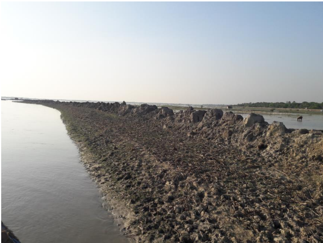
Figure: Dyke of 1 st link canal.
