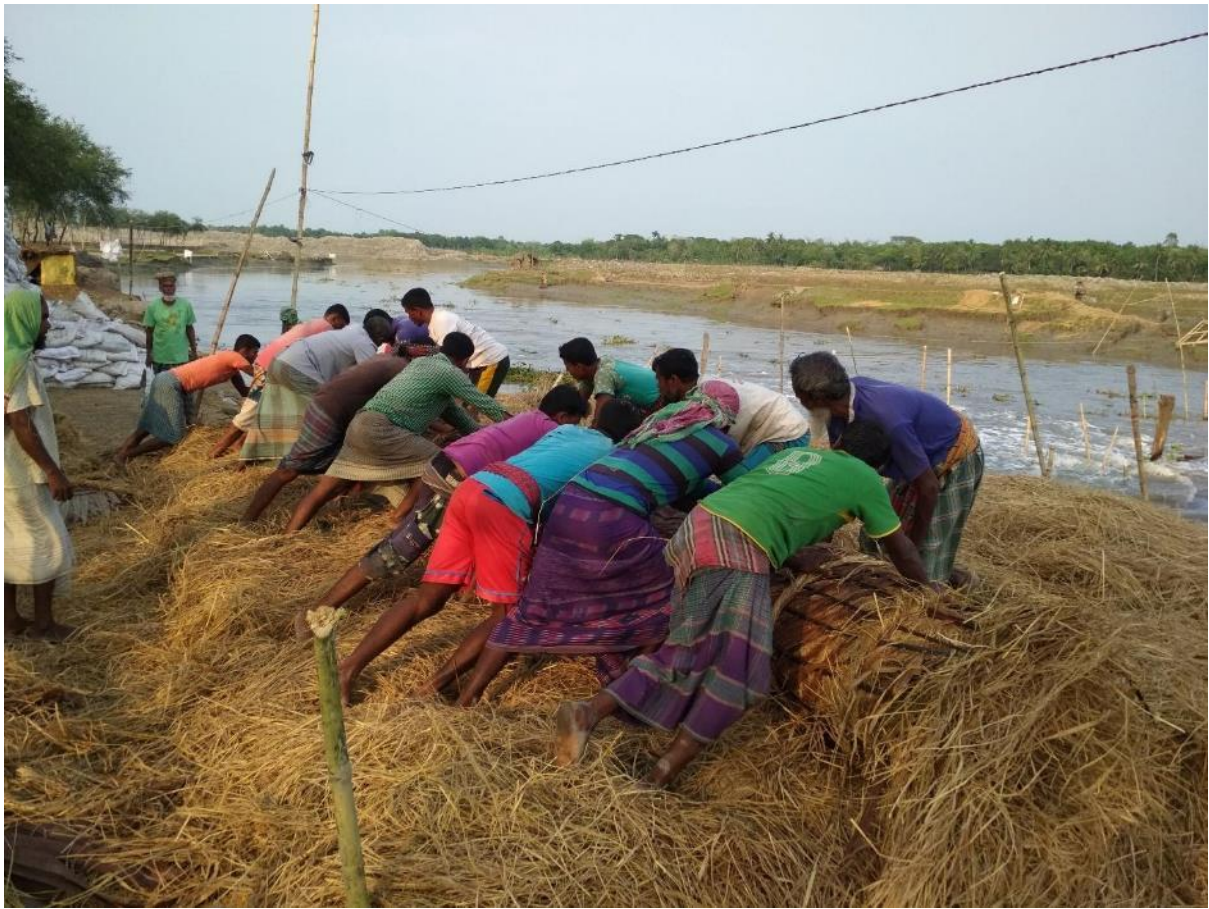
Image 5: Cross dam construction in Kobadak River
