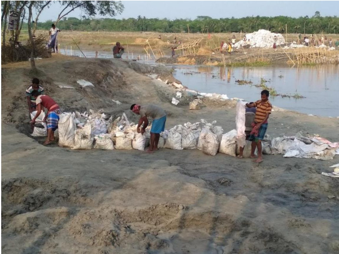
Image 3: Cross dam construction in Kobadak River
