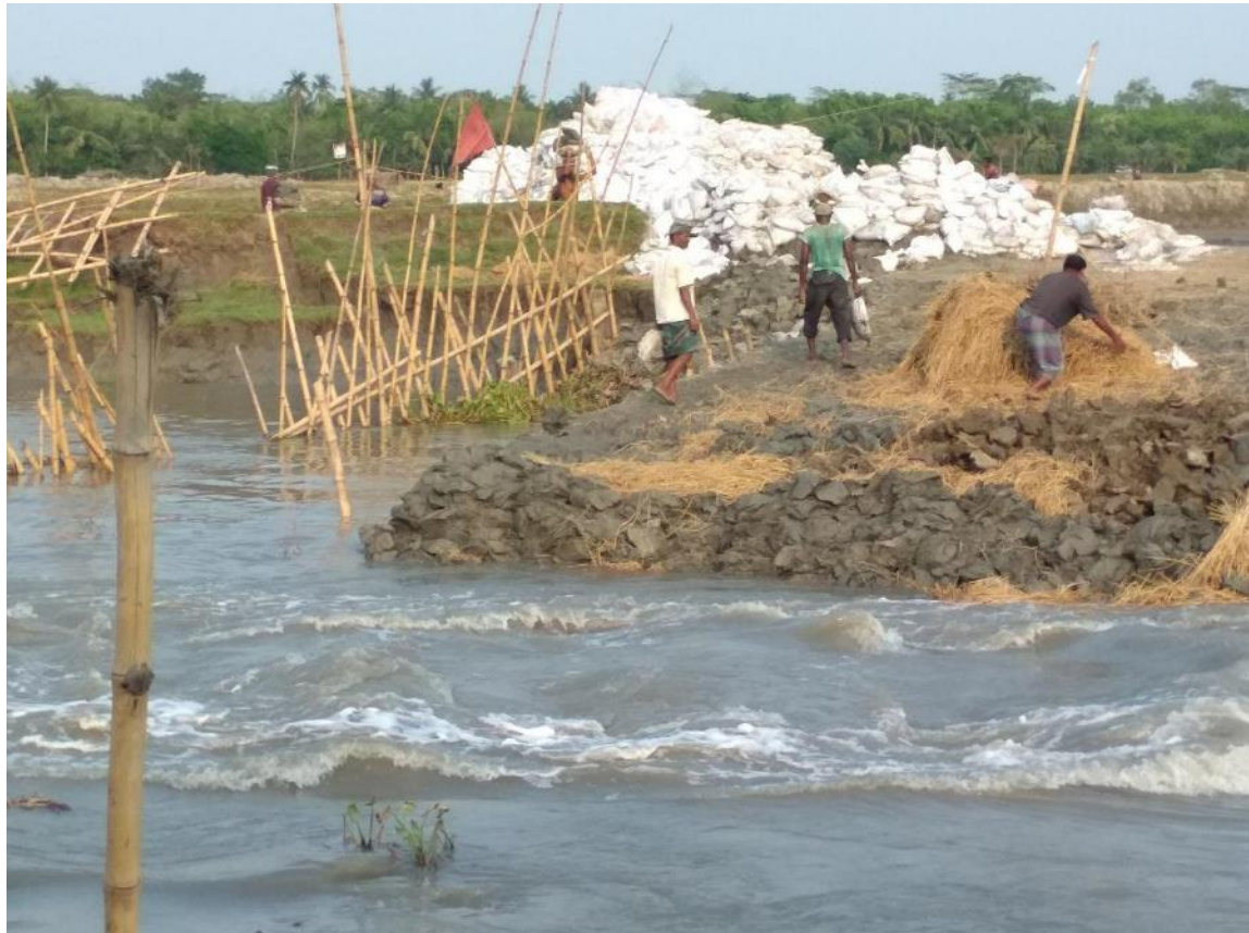
Image 4: Cross dam construction in Kobadak River
