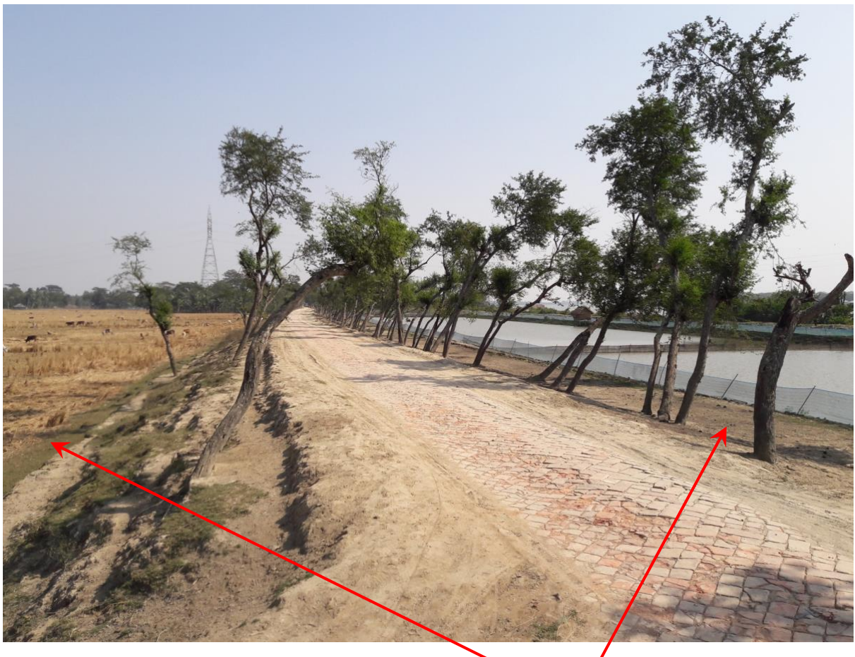
Land Elevation Difference in Polder 30, inside and outside of the polder.
