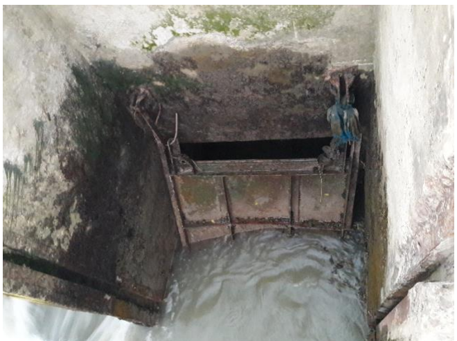
Fully nonfunctional sluiceway in Soabaki (22.572338, 89.779705).
