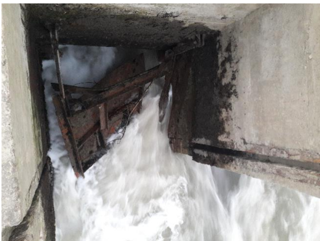
Fully nonfunctional sluiceway in Soabaki (22.572338, 89.779705).
