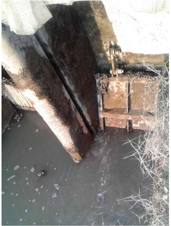
Poorly functioning Sluiceway in the Par Batiaghata (22.729765, 89.468265)
