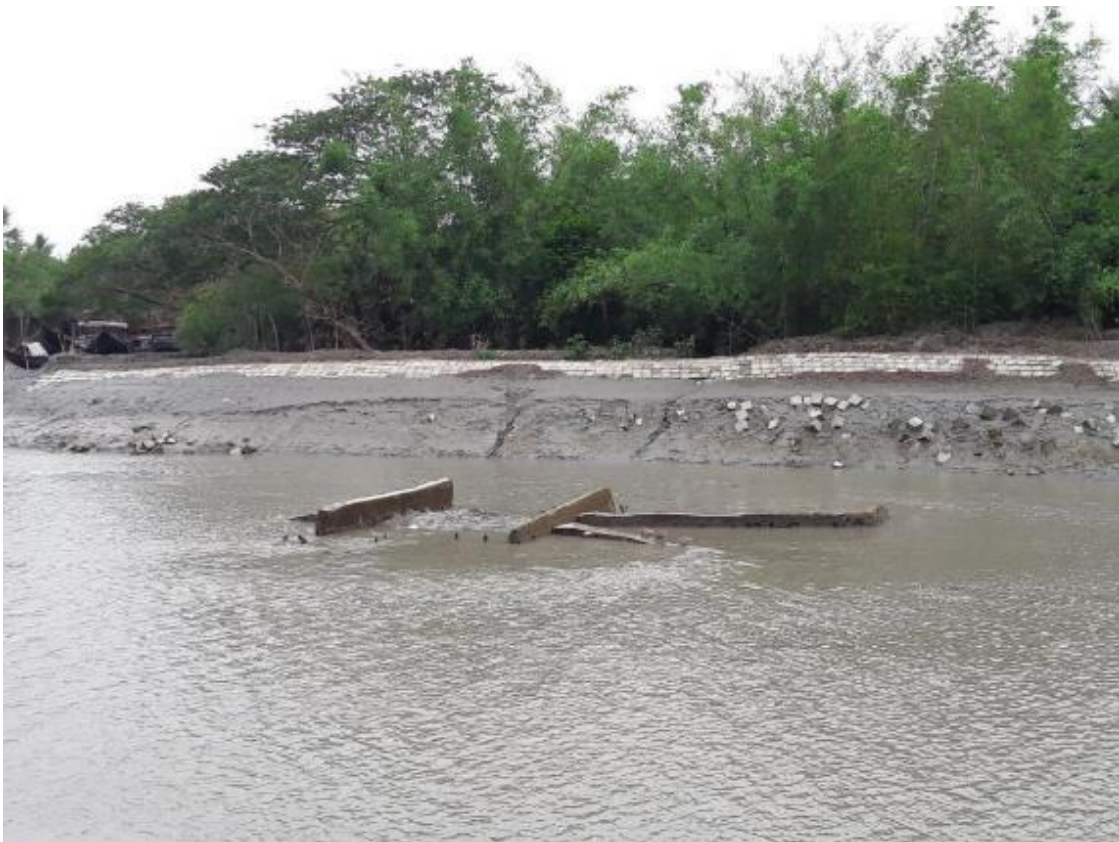
Image 12: Remaining water controlling structure (constructed before TRM) on the link canal
