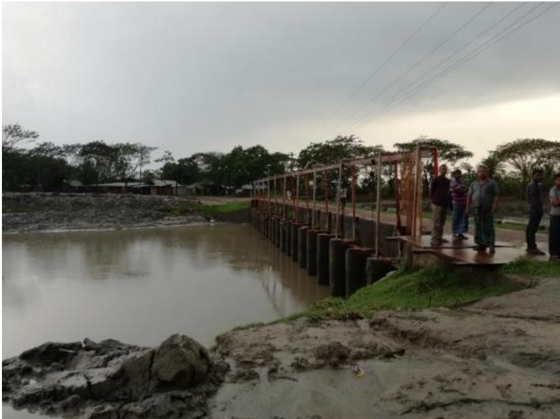
Image 31: Nine vent sluice gate on Bhabadaho River
