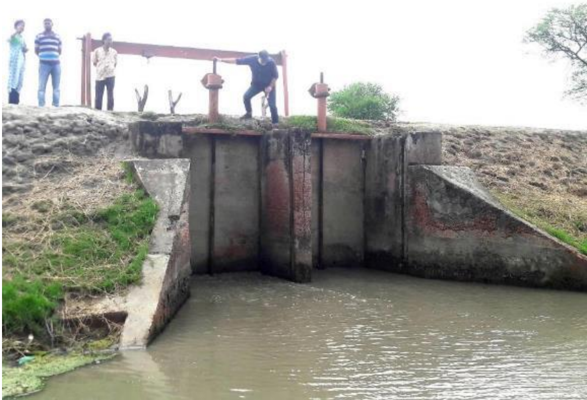
Image 23: Two vent sluice gate in Bhaina
