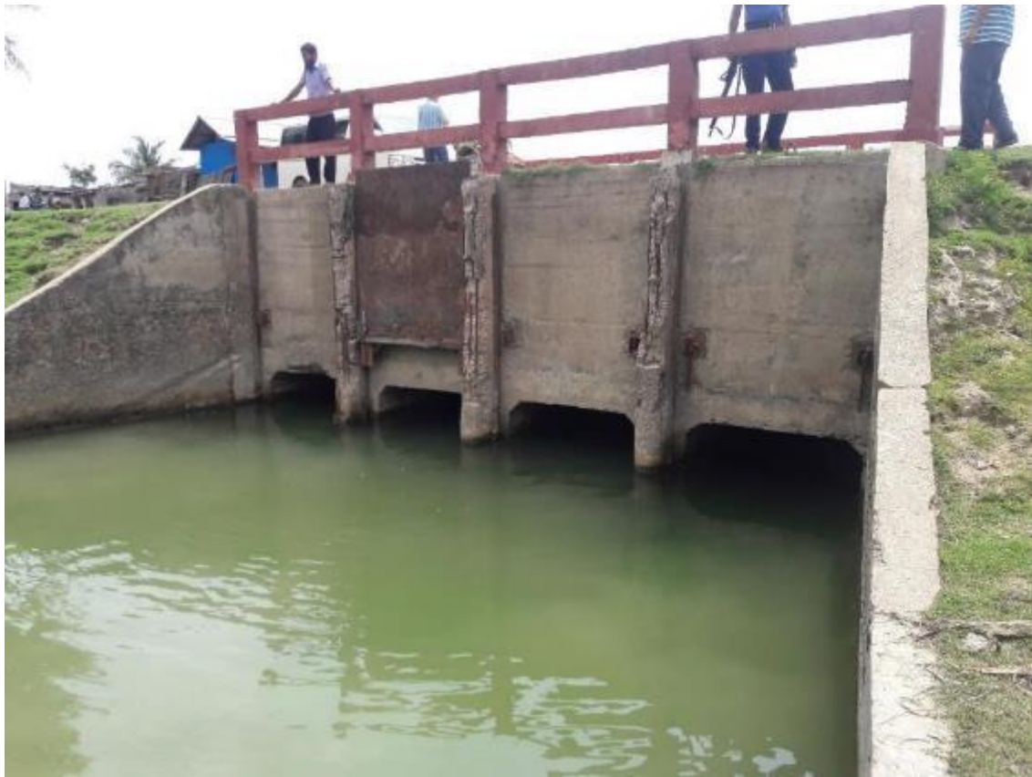
Image 3: Four vent BWDB sluice on Jethua Khal (inner side)
