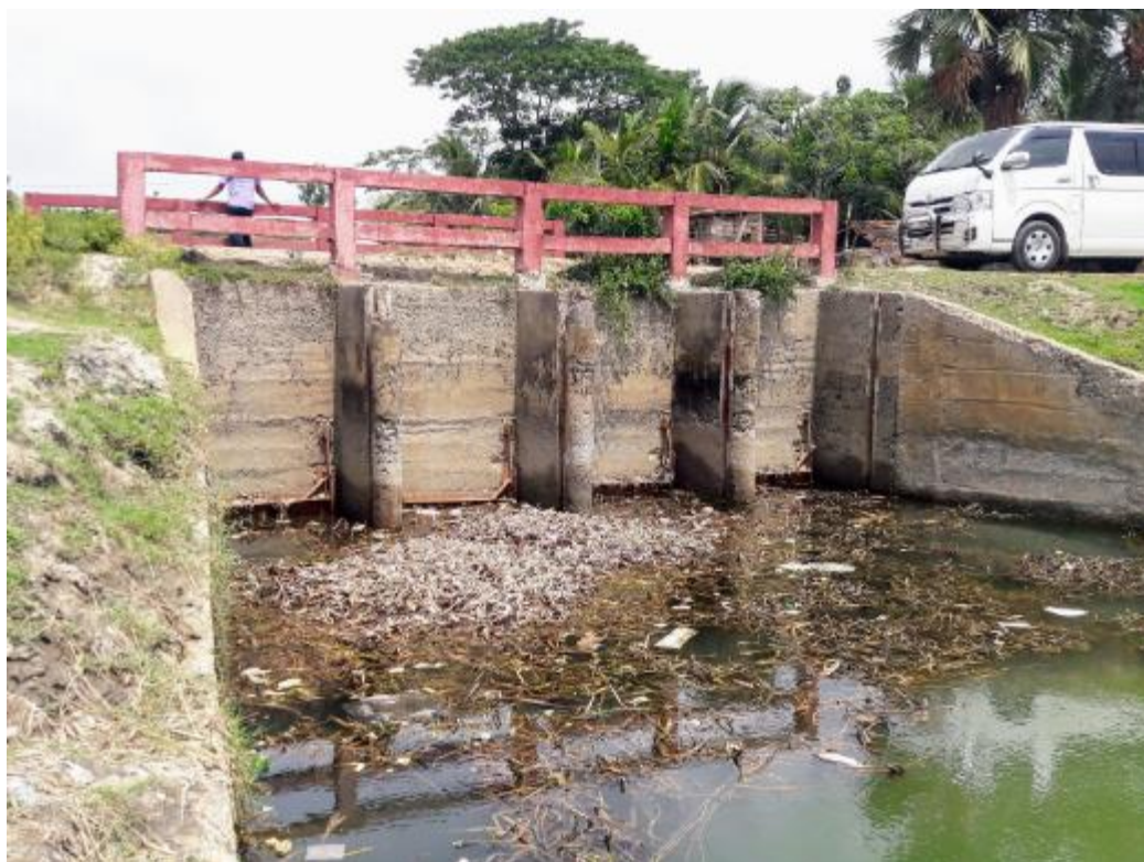
Image 2: Four vent BWDB sluice on Jethua Khal
