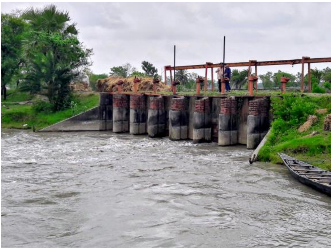
Image 26: Eight vent sluice gate at Khukshia
